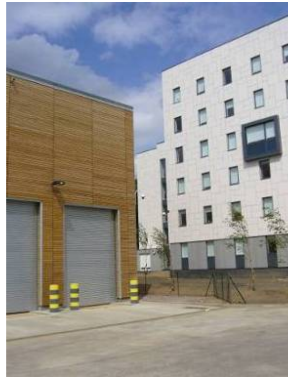
UEA's Biomass Gasification CHP Plant
